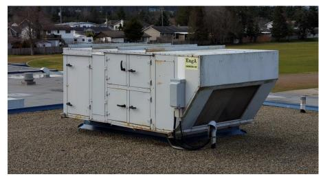
Figure 28: HV11A rooftop unit with DX cooling
