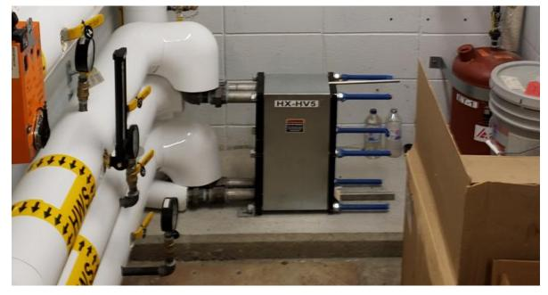
Figure 4: HX-HV5 heat exchanger
