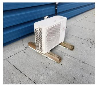
Figure 5: Additional Fujitsu split unit above multi-use area.
