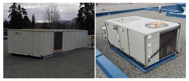
Figure 27: HV2 and HV4 rooftop units with DX cooling
